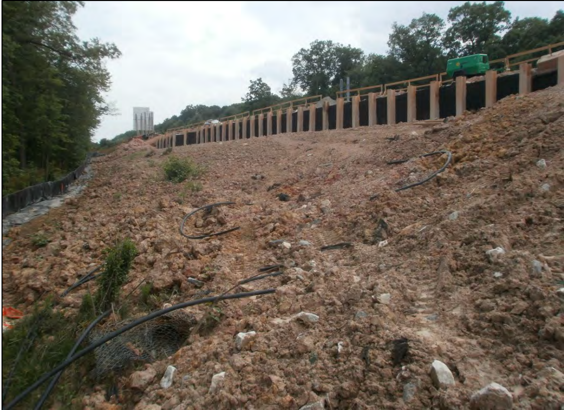
Figure 2-5: Slope stabilization with pile and lagging wall.
