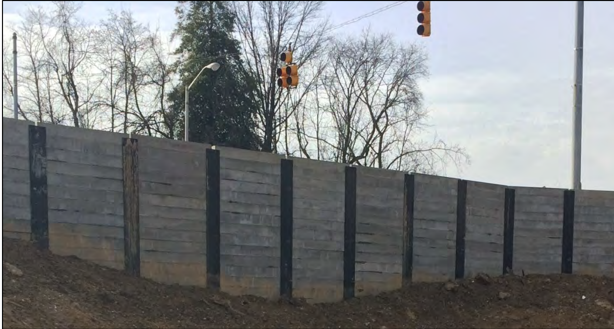
Figure 2-3: Permanent retaining walls: non-gravity cantilever wall.
