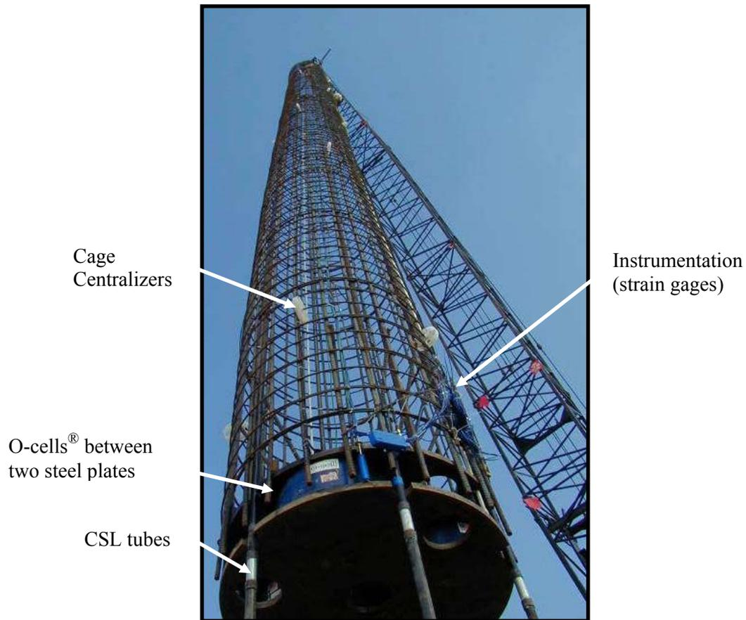
**Figure 9-75. O-Cell<sup>®</sup> assembly attached to a reinforcing cage with other instrumentation.**
