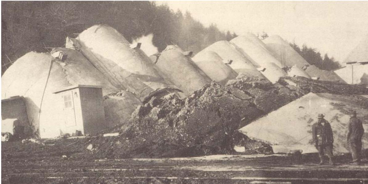
**Figure 8-12. Bearing capacity failure of silo foundation (Tschebotarioff, 1951).**
