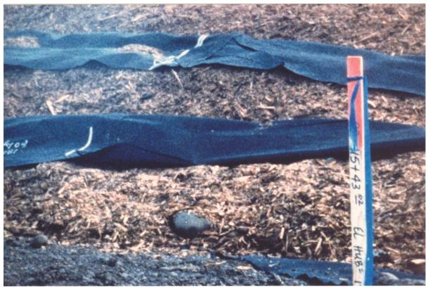
Figure 3-4. Embankment construction with wood fiber.
