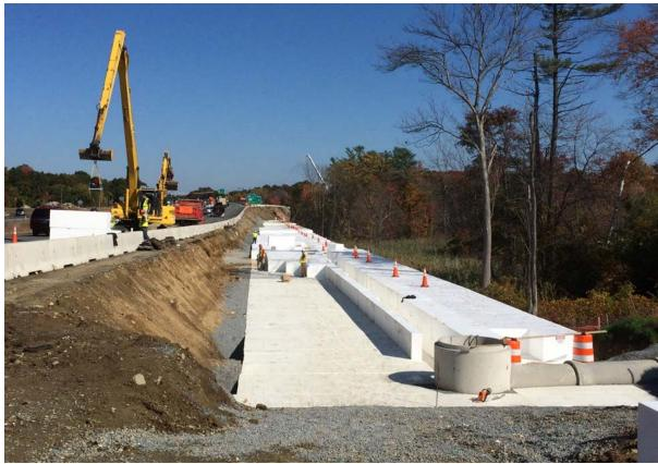
Massachusetts Department of Transportation Figure 3-12. Whittier Bridge EPS block placement on embankment widening.
