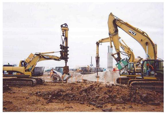
Courtesy Geopier Foundation Company Figure 5-28. Rammed aggregate pier installation.
