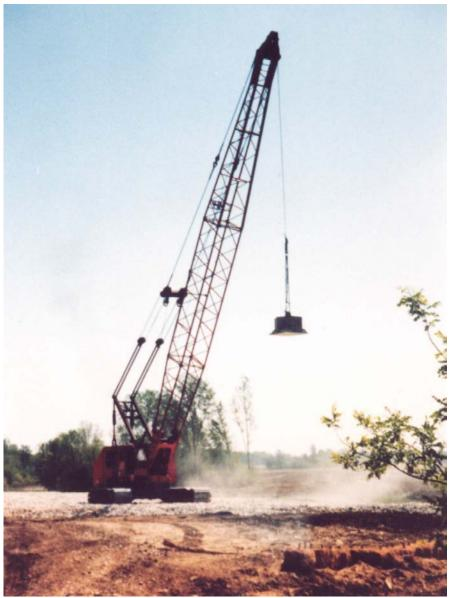
Photo courtesy Bob Lukas, Ground Engineering Consultants, Inc. Figure 4-20. Deep dynamic compaction over a 3-foot layer of crushed rock placed on a landfill.
