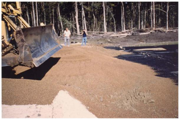
Figure 3-5. Placing expanded clay fill.
