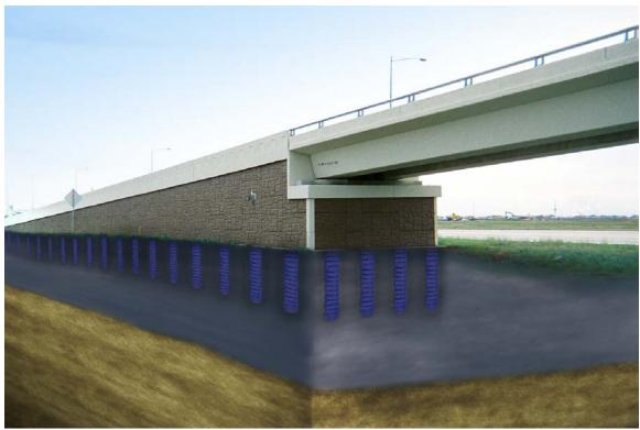
Courtesy Geopier Foundation Company Figure 5-29. Completed MSE wall supported on rammed aggregate piers.
