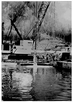
Figure 4-32. Vibrator suspended from a barge-mounted crane.
