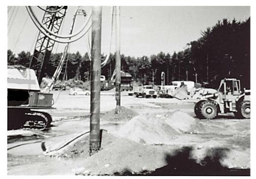
Figure 4-31. Vibrator suspended from a conventional crane.
