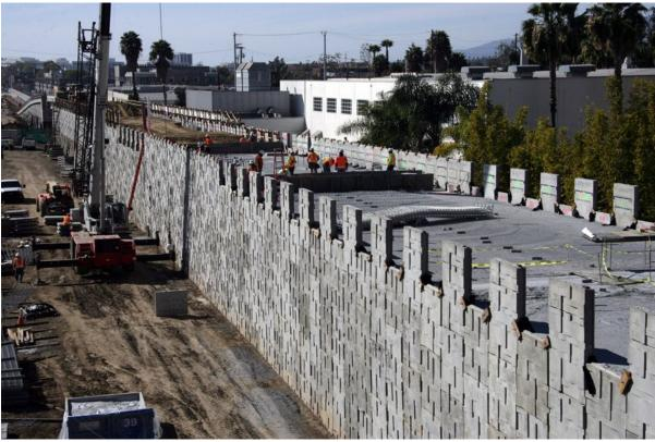
Photo courtesy of MixOnSite USA, Inc. Figure 3-2. Foamed concrete MSE wall backfill for light rail project in California.
