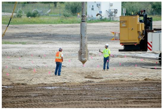
Courtesy of Hayward Baker Figure 4-29. High-powered, probe-type vibrator utilized in vibro-compaction.
