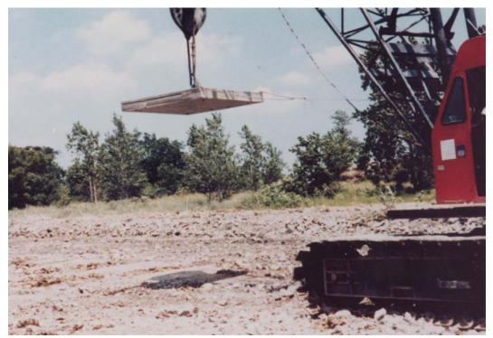
Figure 4-14. Tamper with low contact pressure for ironing pass.
