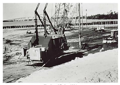
Hussin and Foshee 1994 Figure 4-42. Densification of loose sand backfill during vibro-compaction at Wando Terminal.
