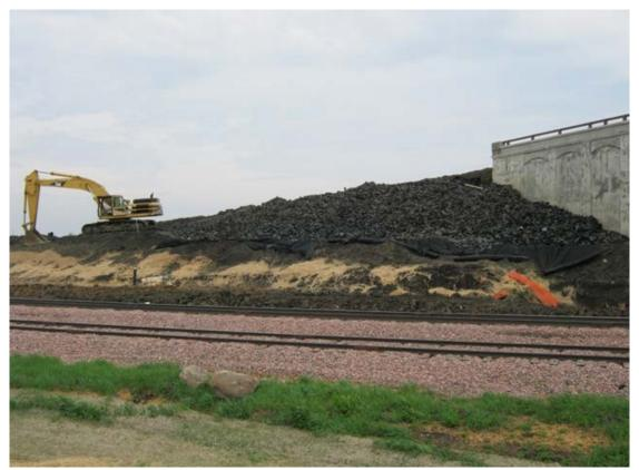
Photo courtesy of Gale-Tec Engineering Figure 3-3. Embankment fill construction with tire shreds in Blue Earth County, Minnesota.
