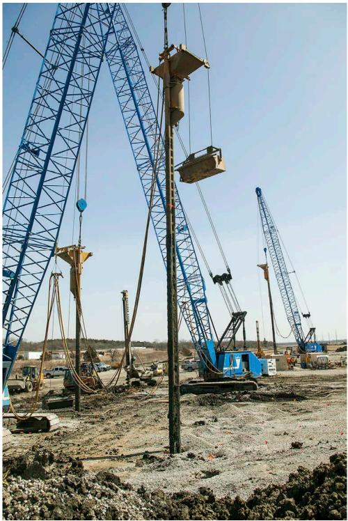
Courtesy Hayward Baker Figure 5-7. Stone column dry bottom feed rig.
