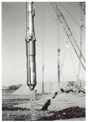
Figure 5-4. Suspended vibrator.
