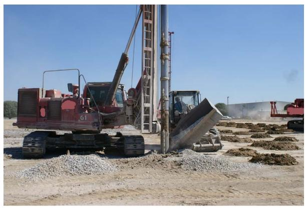
Courtesy Subsurface Constructors Figure 5-9. Top feed vibro rig.
