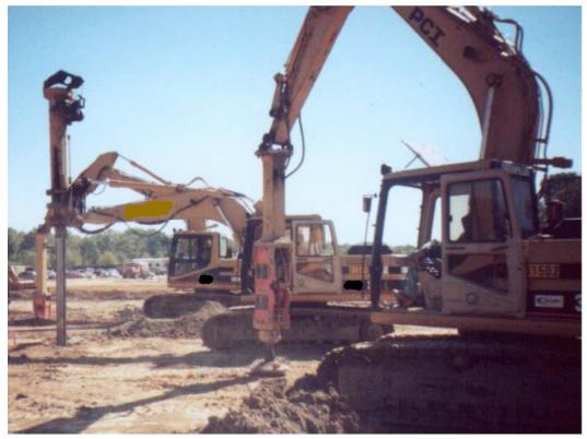
Courtesy Geopier Foundation Company Figure 5-14. Rammed aggregate pier tamper.
