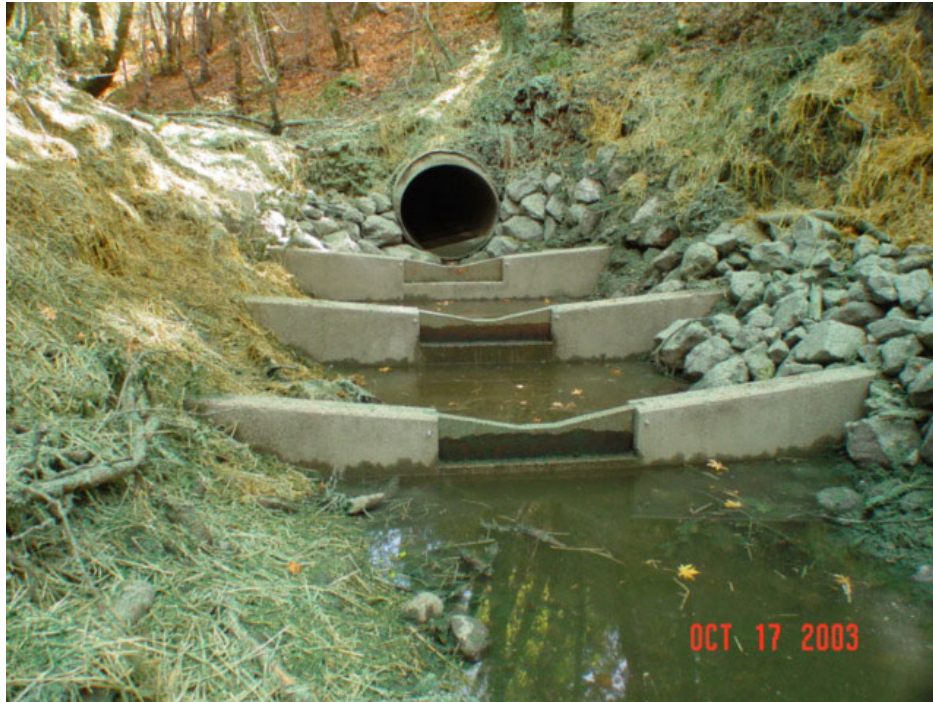
Figure 8.16 Culvert outlet after installation, John Hatt Creek
