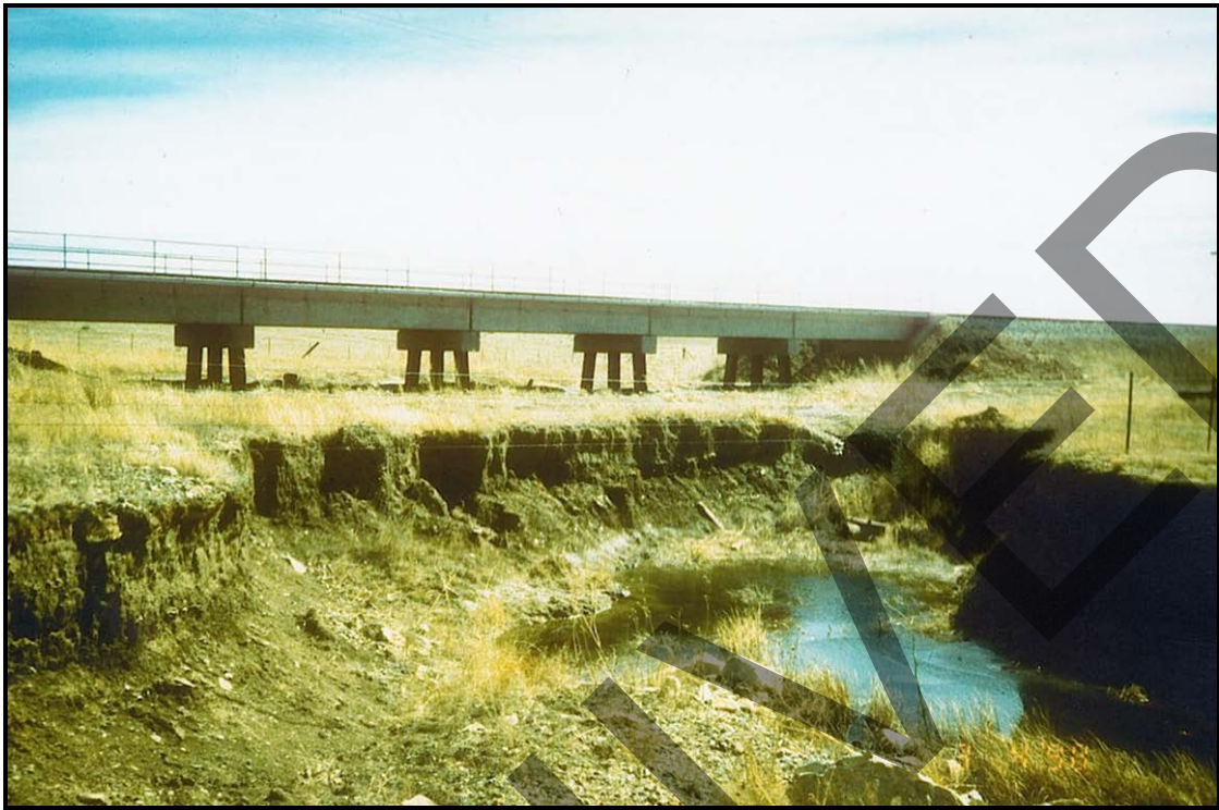
Figure 8.10. Headcut downstream of a bridge.
