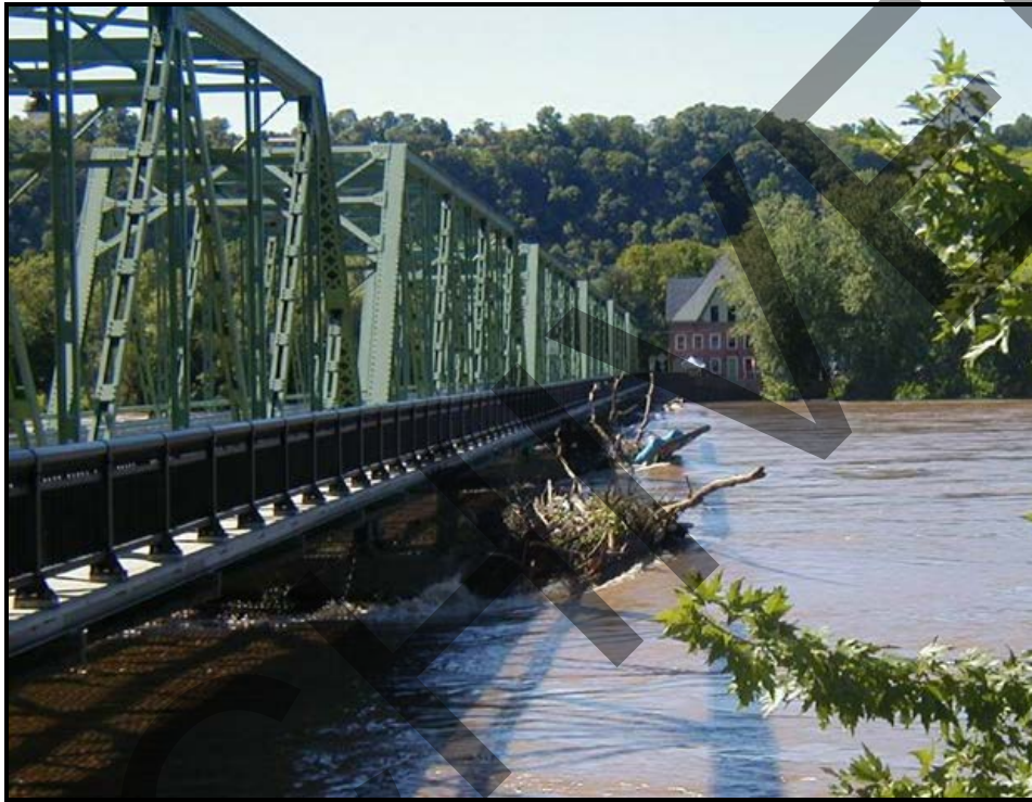
Figure 3.12. An example of debris blockage on piers.
