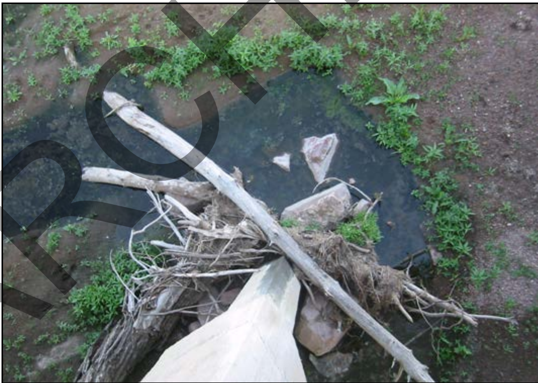
Figure 8.7. View down at debris and scour hole at upstream end of pier.
