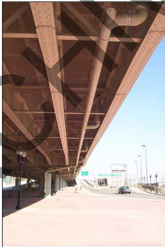
Figure 10.14. Installed underdeck bridge drainage system.
