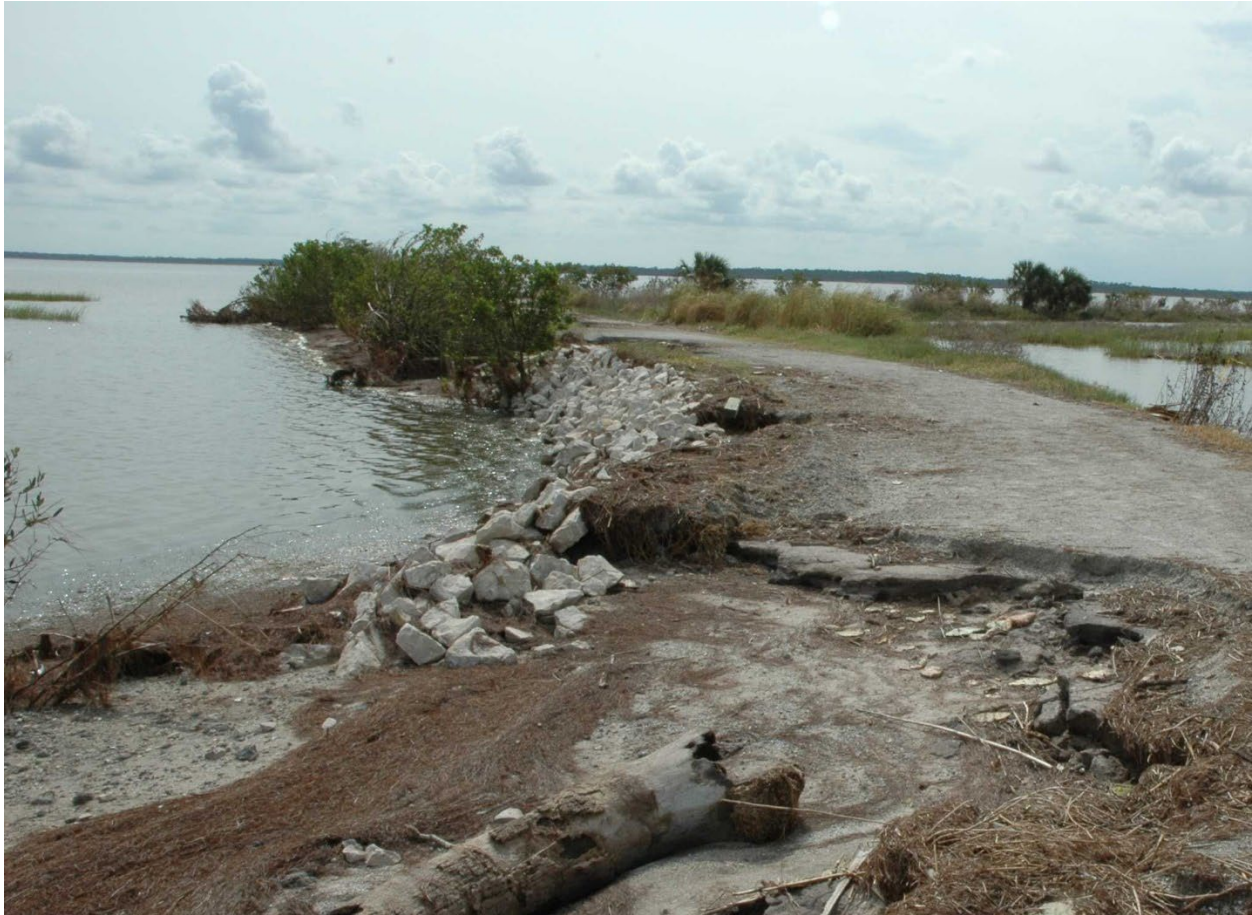
Figure 6. Local roadway damage from Hurricane Jeanne (FHWA photo).
