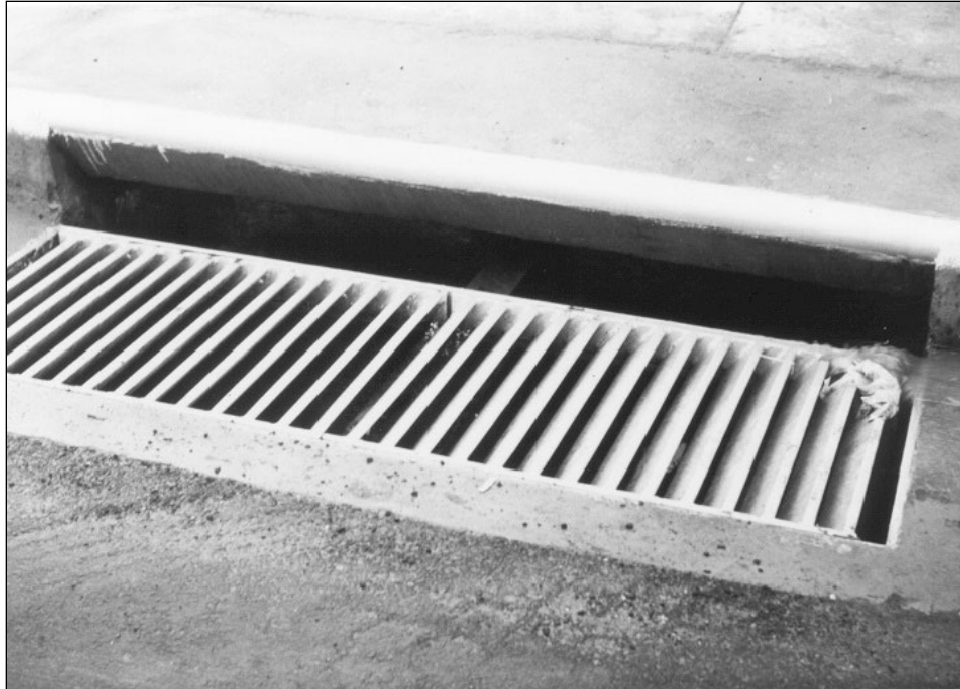
Figure 7.11. Combination curb-opening with 45-degree tilt-bar grate inlet.
