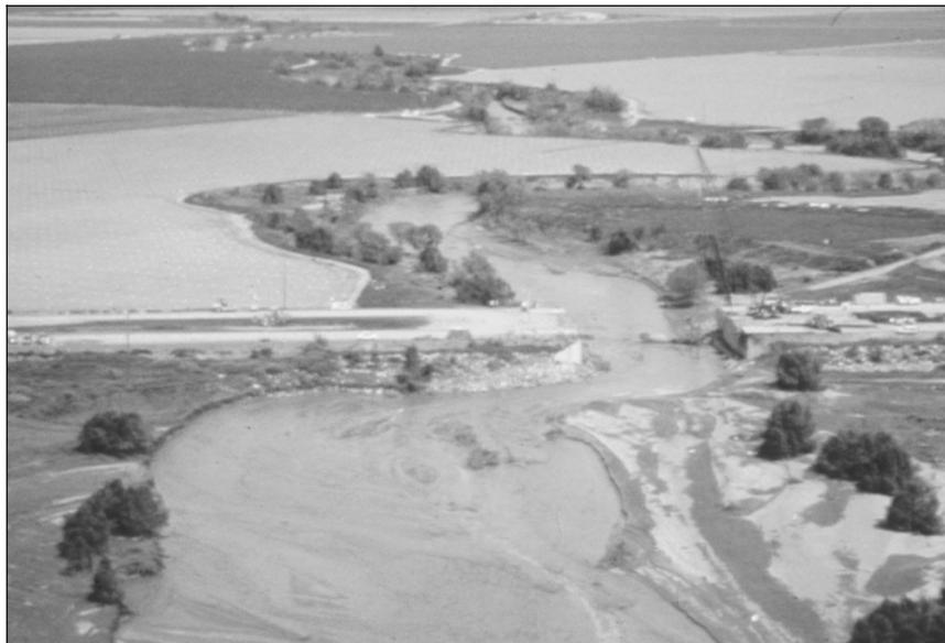
Figure 2.2. Live-bed contraction scour contributed to failure of the I-5 bridges near Coalinga, CA.
