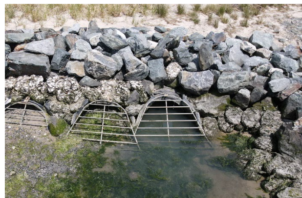
Figure 4. Coastal green infrastructure at Reed Ave to improve drainage and project against flooding (Source: Delaware DOT).
