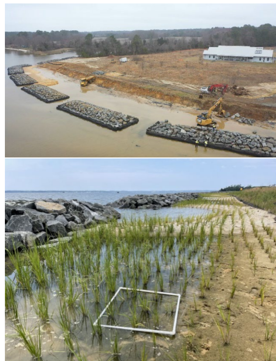
Figure 3. Nature-based solutions projects for shoreline restoration in the Chesapeake Bay, including breakwater in the top picture and vegetation monitoring below (Source: Virginia DOT).
