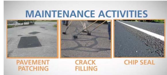
Maintenance activities to keep facilities in good repair do not require accessibility modifications. Examples of pavement maintenance treatments are chip seals, crack filling, and pavement patching.
