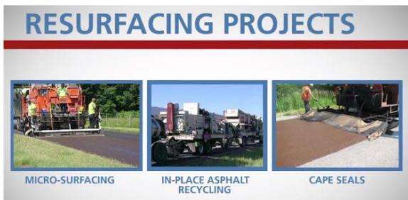
Resurfacing projects are not always simple asphalt overlays. Micro-surfacing, in-place asphalt recycling, and cape seals are
