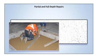
In cases where deterioration exists below the upper third of the slab, agencies may elect to perform a full-depth repair or slab replacement. While the timely and appropriate application of this treatment can extend pavement performance beyond ten years, it is costly.
