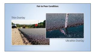
Ultrathin overlay materials consist of a designed asphalt and small stone mixture that is prepared in a plant and hauled to the site. Following the application of a thick layer of liquid asphalt tack coat, crews apply less than 1 inch of the ultrathin material mixture.
