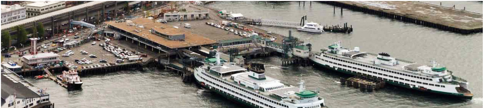
The Seattle Multimodal Ferry Terminal at Colman Dock
