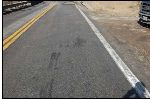
DSC8.JPG - View of Vehicle #1 left front pre-impact tire mark end
