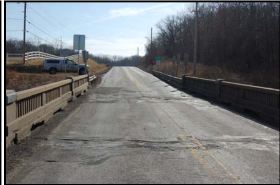
DSC14.JPG - View of crash scene, looking east
