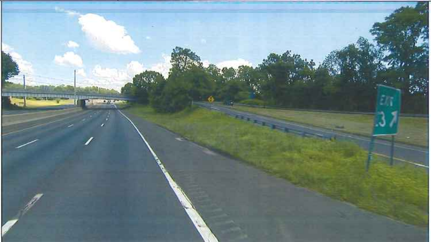
Connecticut -Route I-95 Northbound at Mile Post 24.26 – Photolog Picture of system taken prior to accident
