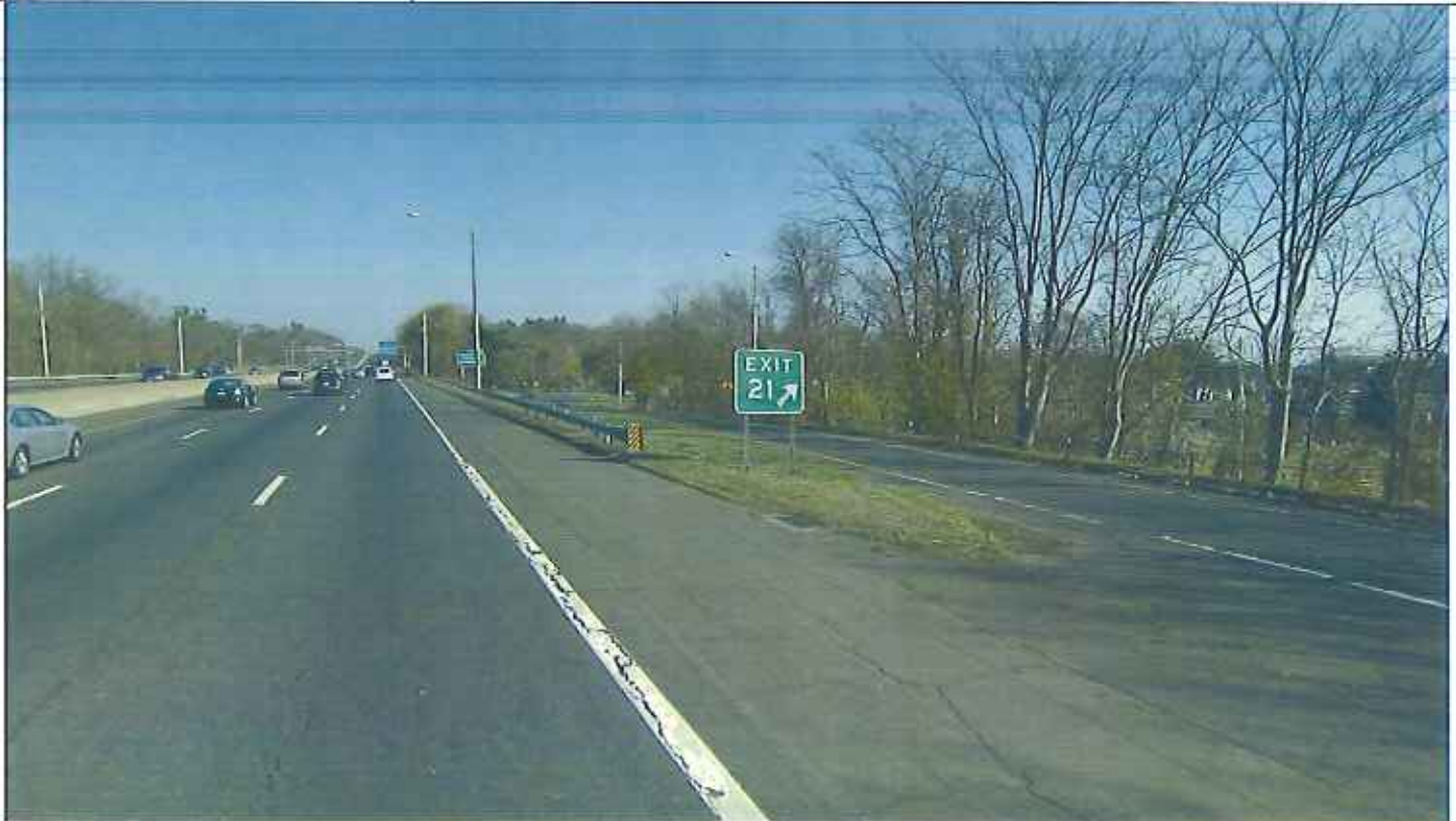
Connecticut -Route I-95 Northbound at Mile Post 24.26 – Photolog Picture of system taken prior to accident
