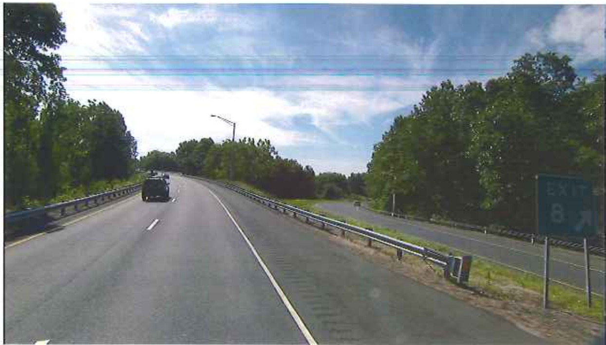
Connecticut -Route 2 Eastbound at Mile Post 5.36 – Photolog Picture of system taken prior to accident
