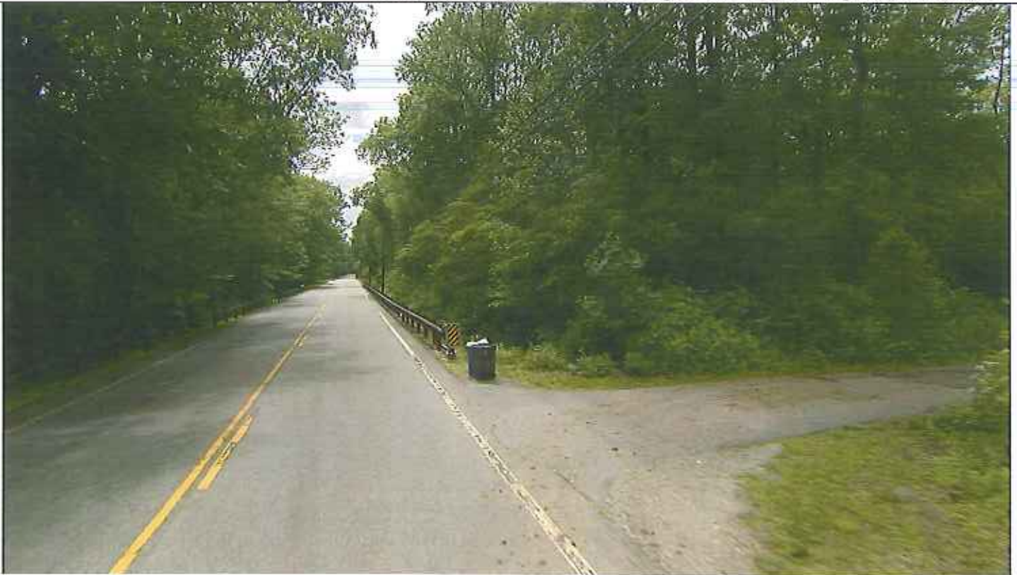
Connecticut -Route 184 Westbound at Mile Post 9.16 – Photolog Picture of system taken prior to accident
