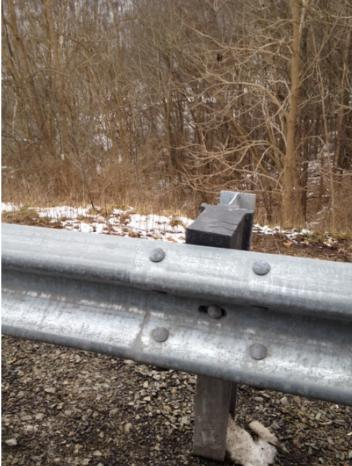
Significant photos— Holes in weak post bottoms No holes in strong post bottoms 4 slots in rail just after ET for cable ET+ =4 rails each 12' with 8 bolts overlap 1' 50 feet of rail + ET Posts are 4 feet apart-police report says "6 posts And 3 rails damaged". Doug, Green acres guy, said end cut off with blow torch. Thought it was 2<sup>nd</sup> or 3<sup>rd</sup> rail still in ET. ET Plus sticker on top of ET
