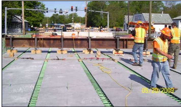
Fig. 12 Adjusting the Girder Camber Prior to Casting the UHPC Joint Fill
