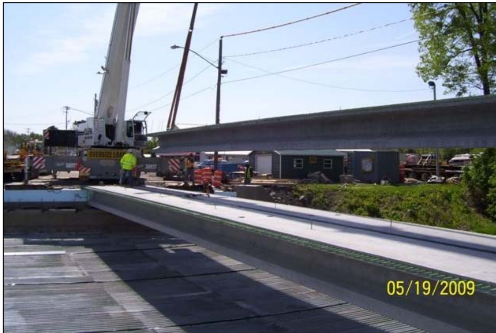
Fig. 11 Installing the side-by-side Deck Bulb-Tees
