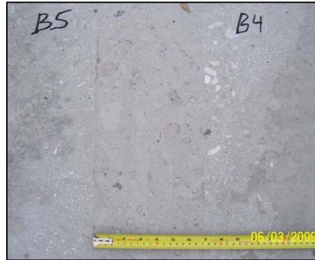
Figure 15 Close-up of a ground Joint Fill and side-by-side Deck Bulb Tees
