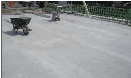
Fig. 16 Top view of bridge deck before applying asphalt overlay. Showing UHPC Joint Fill and side-by-side Deck Bulb-Tees.
