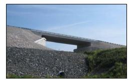
Hawk Lake Bridge, Ontario (2008) is another successful Ductal<sup>®</sup> Joint Fill project with an advanced precast bridge deck system. Advantages and benefits include: simplified fabrication and installation processes, superior freeze/ thaw resistance, extremely low porosity, improved flexural strength, superior toughness with resistance to harsh climates and continuous flexing from truck loadings across the joints.
