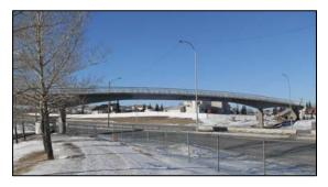
\*The **Country Hills Pedestrian Bridge**, Alberta (2008) has a 33.5 m Ductal<sup>®</sup> drop-in girder. This 49 m clear span bridge crosses over 6 lanes of traffic, providing the two adjacent communities with an aesthetically pleasing, durable curved-linear link. This is the first pedestrian bridge project where Ductal<sup>®</sup> was batched in a ready mix truck
