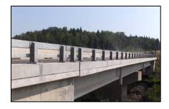
The **Current River Bridge**, Ontario (2007) utilized Ductal<sup>®</sup> Joint Fill for precast curb sections under bridge railings.
