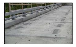
The **Rainy Lake Bridge**, Ontario (2006) is the world's first Ductal<sup>®</sup> Joint Fill ("JS1000") project; part of an innovative field cast joint solution for a bridge superstructure/precast deck panel system specially developed for the Ministry of Transportation of Ontario. Through its design, testing and construction, this project validated a precast bridge deck with a 200 mm wide joint (conventional design is 600 mm wide) and led the way to other, repetitive joint fill projects.
