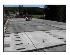
The following bridges, "Buller Creek" and "Log River", were completed for the Ministry of Transportation of Ontario (MTO) in 2009. Each bridge is constructed with precast concrete and joined together with Ductal<sup>®</sup> Joint Fill -- resulting in extremely durable, advanced bridge deck systems that will last, through harsh climates and heavy traffic loads for many decades ahead.
