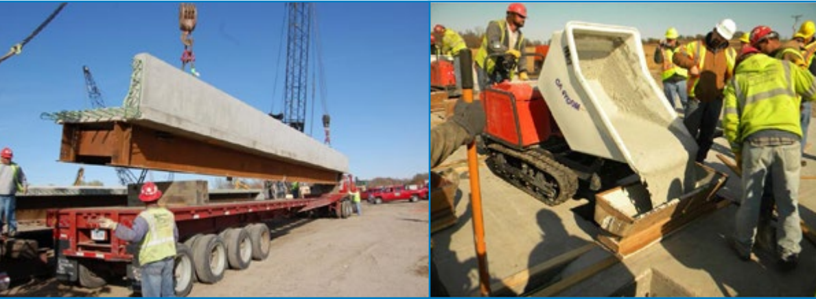
Left: Crews used prefabricated modules to shorten closure time and minimize traffic impact on an Iowa bridge project. Right: Workers poured ultra-high-performance concrete in the joints between the modular superstructure units.
