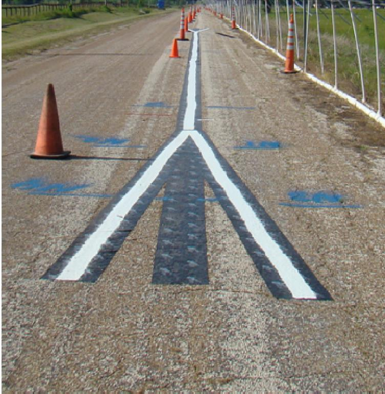
**Figure 8.** Experimental pavement marking applied to black polymer film to allow easy removal of the test markings after completion of the Task 2 experiment
