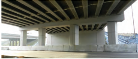
Completed precast bent system demonstration project bridge over I-5 in Washington State.
