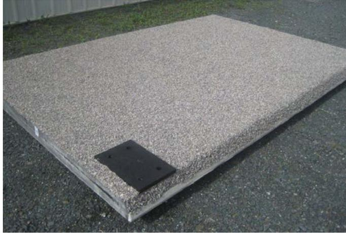
Figure 7. Photo. Adhesive and stone are applied for course 1 of the wearing surface. (The black rectangle is a bearing pad for the bridge railing post.)
