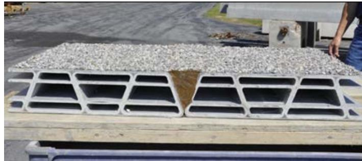
Figure 64. Photo. Panel-to-panel field joint.
