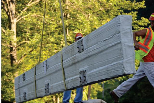
Figure 1. Photo. Ice shield constructed by XC Associates.
