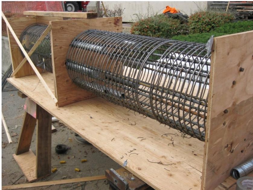
Figure 155. Photo. Column segments for specimens SF-1 and SF-2 were match-tied at a bridge construction site in the City of Redmond.
