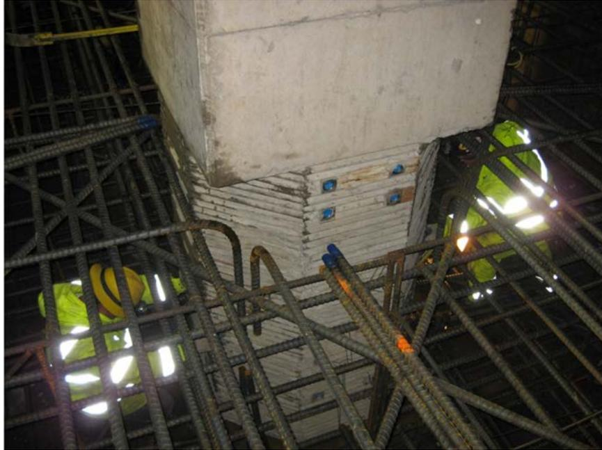
Figure 3. Photo. Earlier form of the socket connection used by the City of Redmond over Washington State SR 520, as originally used.
