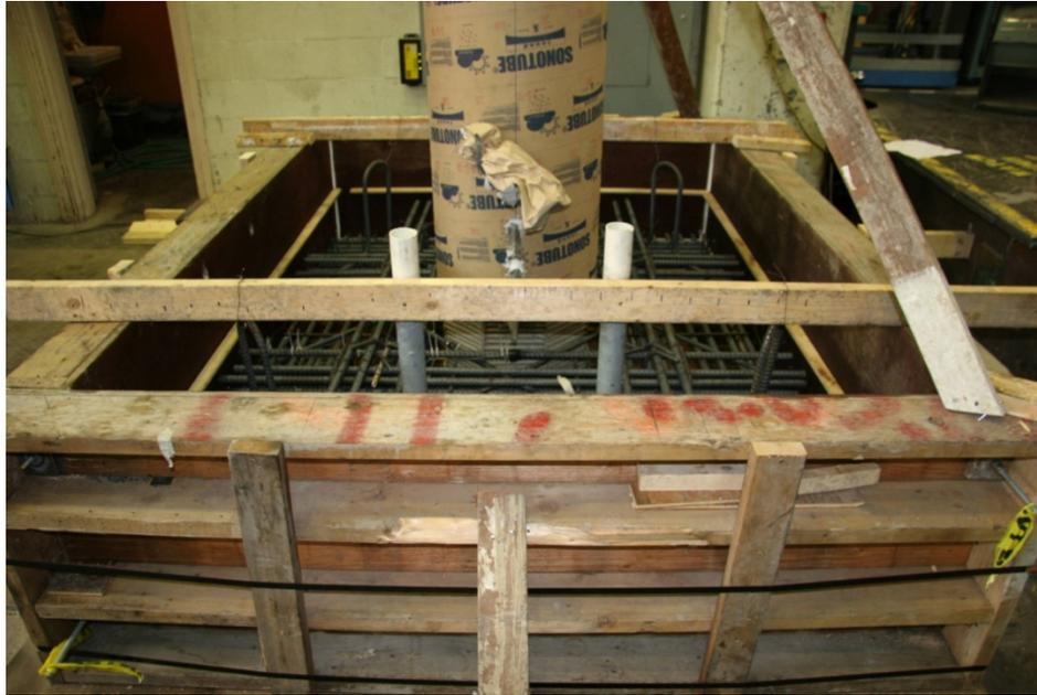
Figure 161. Photo. Specimen SF-3 column inserted into footing that is ready to cast.
