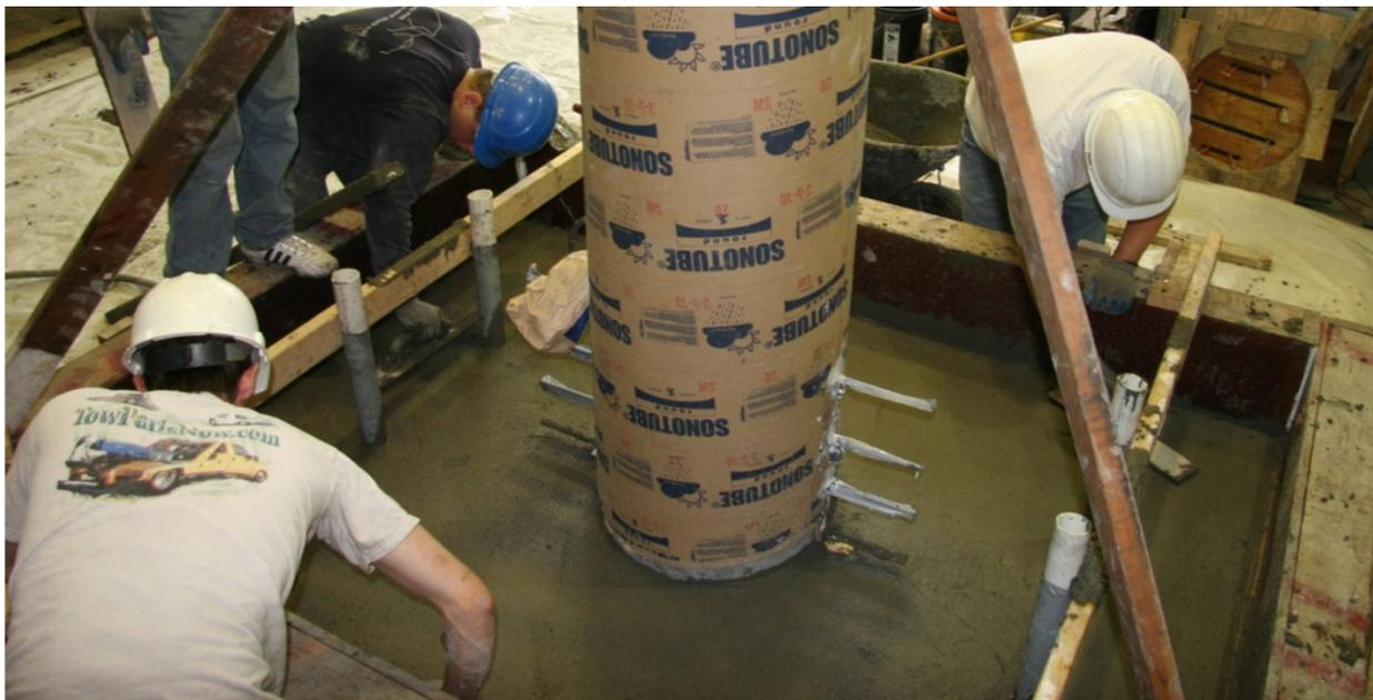
Figure 162. Photo. Specimen SF-3: finishing the footing surface.
