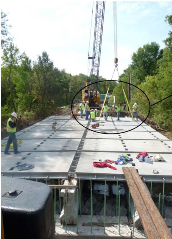
a) Installation of UHPC waffle deck panels
