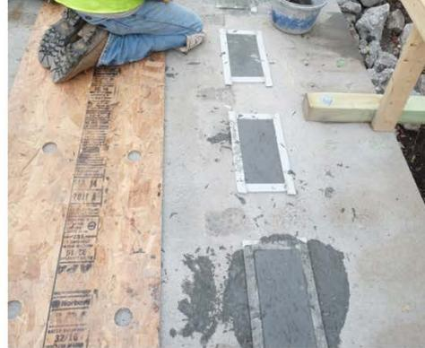
**c) Shear pocket with UHPC joint fill**
