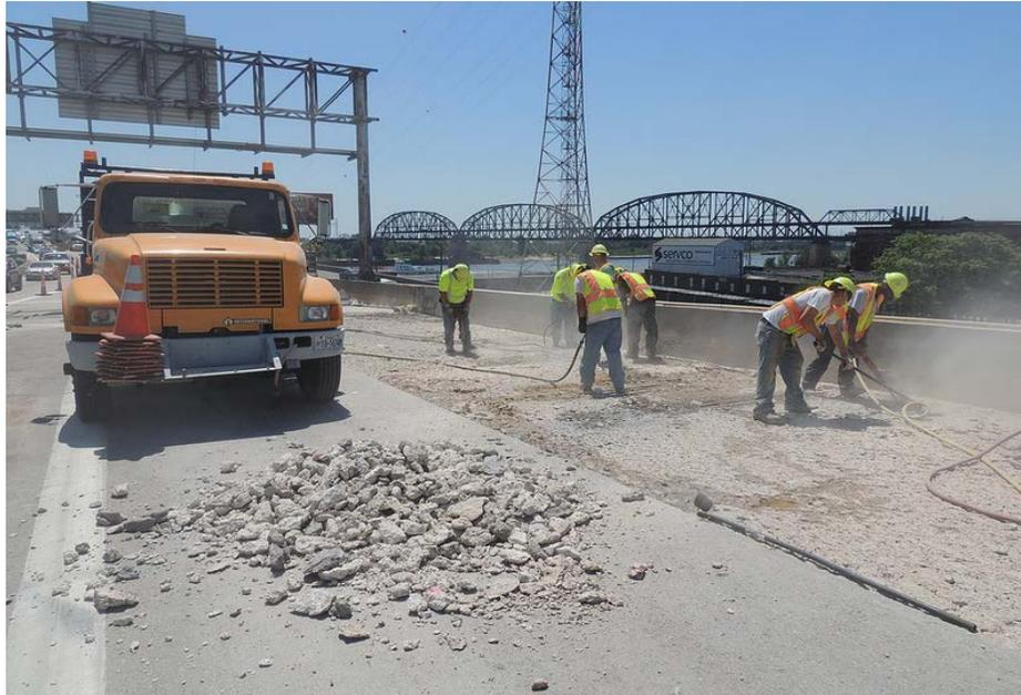
Figure 67. Photo. Jackhammering deck sections prior to removal.
