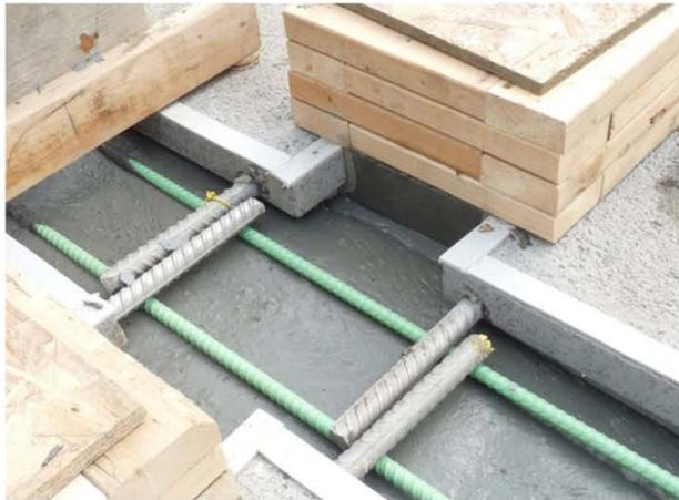
**d) Longitudinal joint filled with UHPC**
