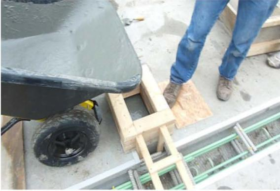
**a) Pouring UHPC joint fill into shear pocket using a wheel barrow**
