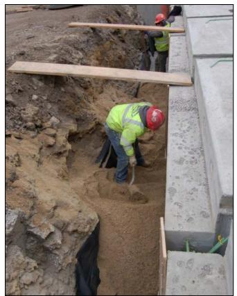
Figure 15. Workers spread granular backfill behind an abutment.
