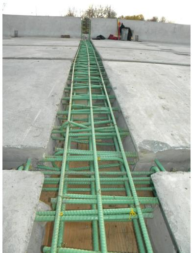
Figure 18. Pier joint reinforcement.
