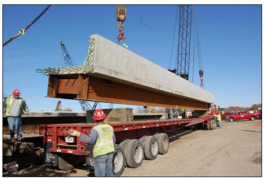
Figure 8. Lifting an exterior module into place.
