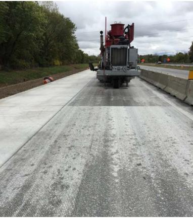
Figure 12. Photo. Application of NGCS – second pass.
