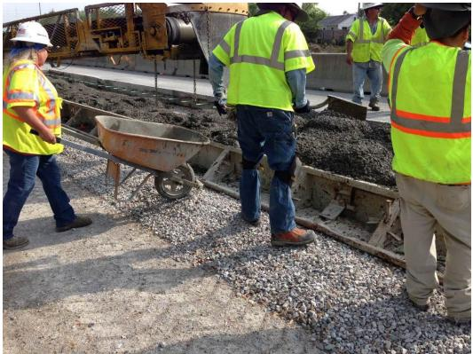
Figure 8. Photo. Placement of fresh concrete.
