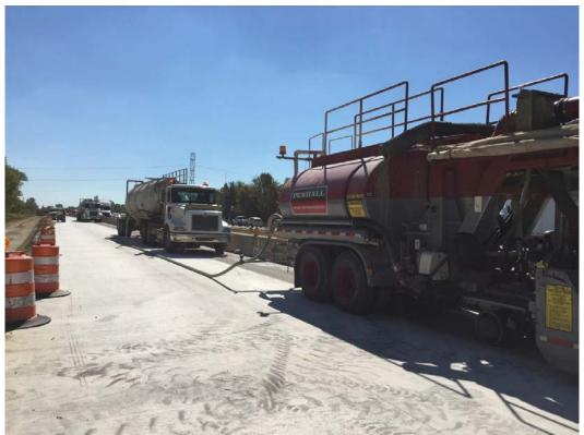
Figure 10. Photo. Application of NGCS – first pass.
