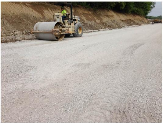
Figure 6. Photo. Subbase preparation for concrete paving.
