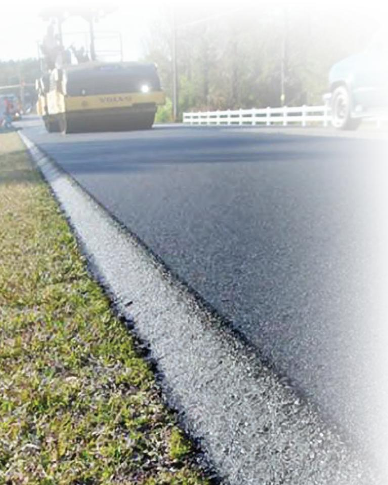
The Safety Edge™ concept originated at the Texas Transportation Institute in 1981, when a team led by Dr. Don Ivey found that a tapered transition between a paved road and an unpaved shoulder helped errant vehicles whose wheels drop off the pavement edge maintain control as they reenter the travel lane. But after the research was done and the papers were written, the idea languished, recalled Frank Julian, safety engineer at FHWA's Resource Center. "It never really got implemented," he said.
