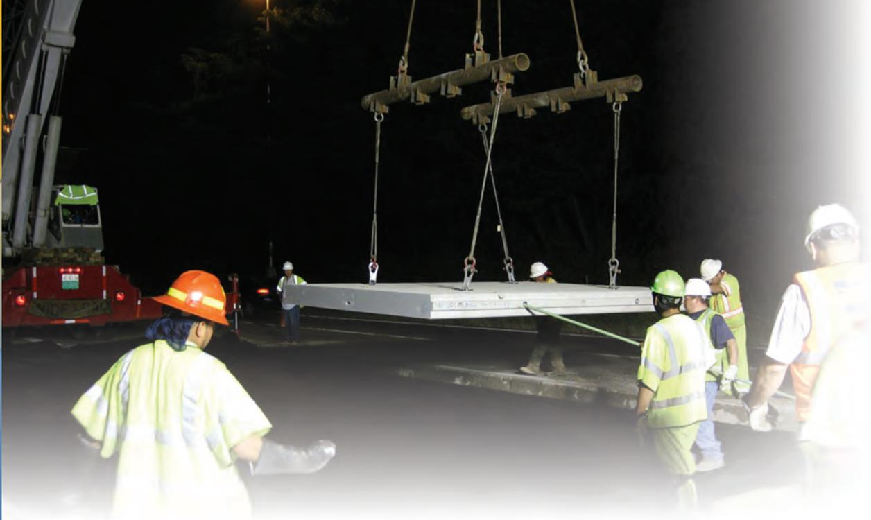
pavement panels reduce traffic congestion, make the construction process safer and increase highway durability. They're particularly useful on high-volume roads where quick repairs are essential to minimize major traffic disruption and extensive user delays.
