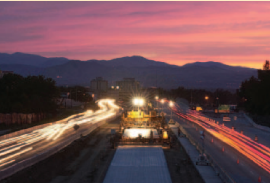
Night paving on the Transportation Expansion Project, I-25 in Denver
