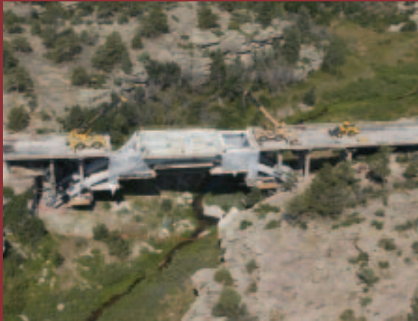
Castlewood Canyon Bridge on SR 83 south of Frantown
