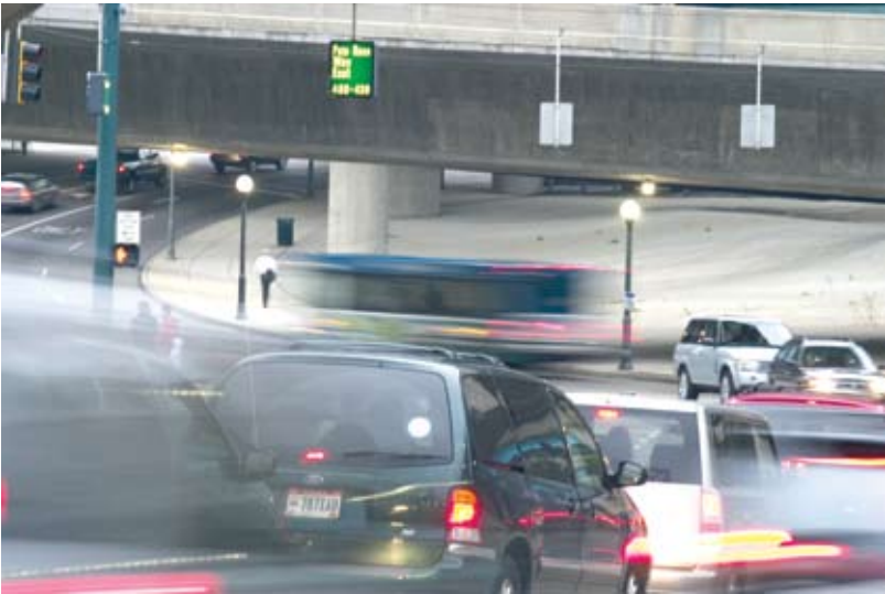
Off-ramp intersecting with Pete Rose Way, Cincinnati, OH.
