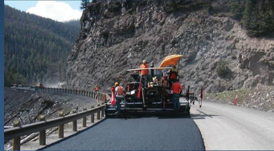
*Lower temperatures for warm mix asphalt are environmentally friendly*
