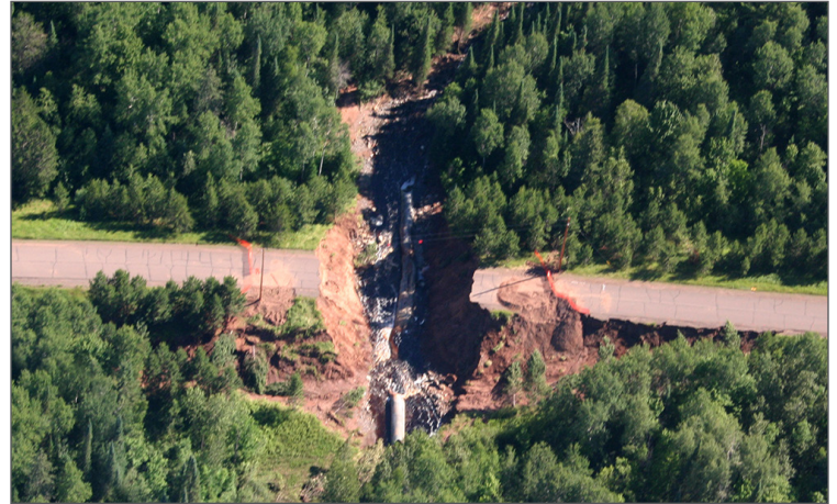
Floodwaters damaged the culvert and washed out more than 100 feet of road at a creek crossing on the Fond du Lac Reservation in Minnesota during June 2012. (Photo courtesy: Central Federal Lands Highway Division)
