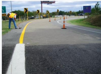
**FIGURE 2:** HFST at horizontal curve
