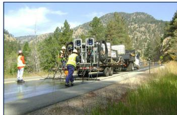
**FIGURE 3:** HFST installations – by hand and by machine
