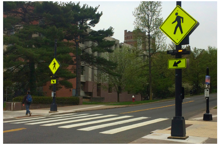
Mid-block pedestrian crossing location with Rectangular Rapid-Flashing Beacons (RRFB).
