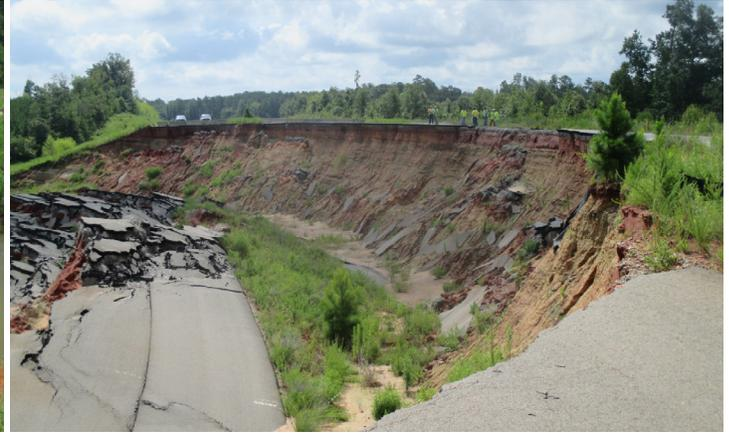
Groundwater conditions missed during geotechnical exploration are a frequent source of problems.
