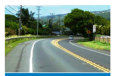
Roadway departure countermeasures applied at this curve include lane separation to prevent head-on collisions, raised pavement markers for visibility, widened shoulders, and a guardrail.
