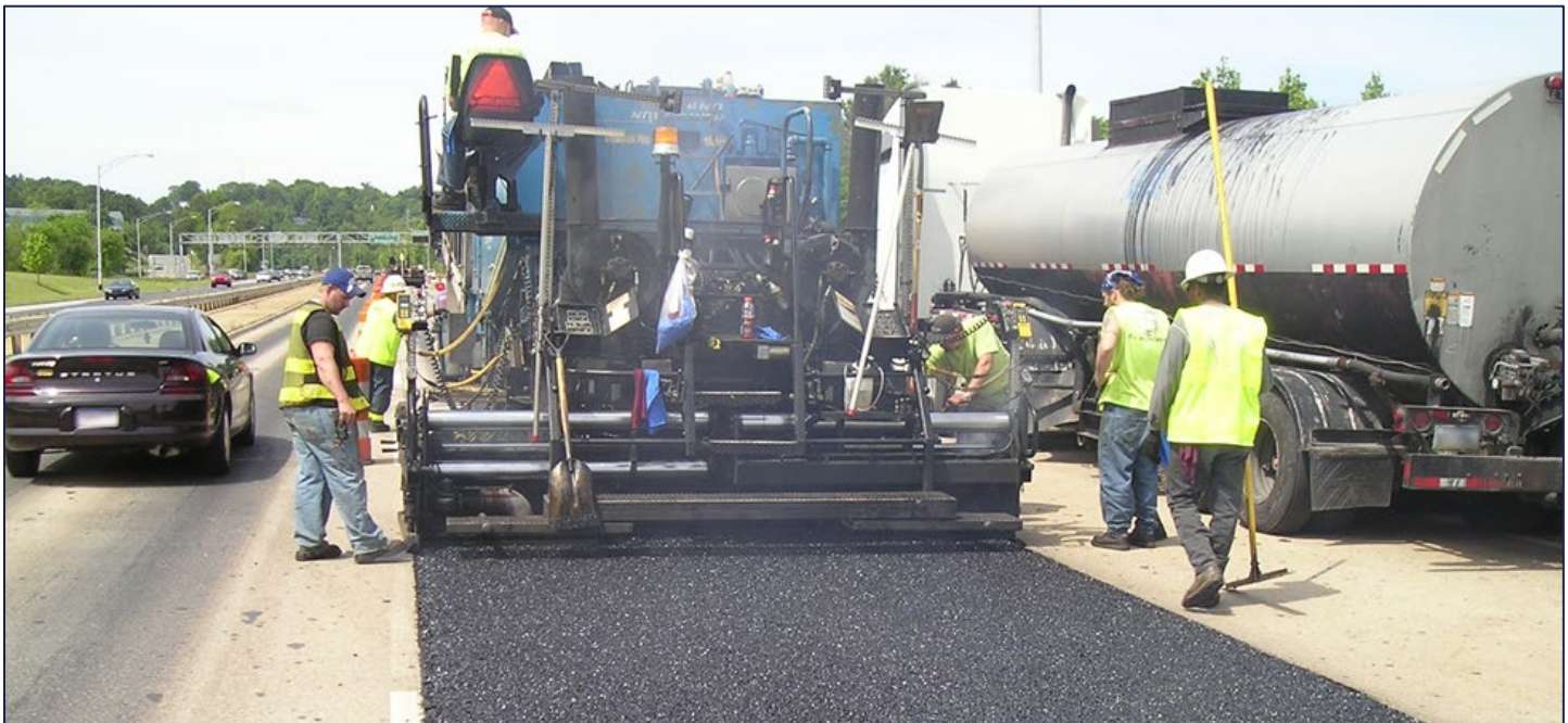
Crews place ultra-thin bonded wearing course. Source: National Center for Asphalt Technology
