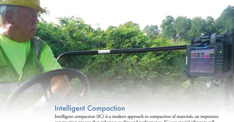
Intelligent compaction (IC) is a modern approach to compaction of materials, an important construction process that enhances quality and performance. IC uses special vibratory rollers equipped with accelerometers, a continuous measurement system, GPS-based mapping, and an onboard computer reporting system. The EDC2 technology initiative will focus on expanding IC use nationwide as a cost-effective way to accelerate highway pavement construction and improve roadway quality.
