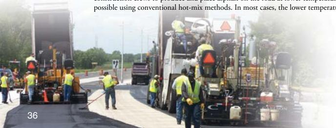
in cost savings and reduced greenhouse gas emissions because less fuel is required to achieve and maintain the temperatures for WMA paving. WMA also has the potential to extend the construction season, enabling agencies to deliver projects faster.
