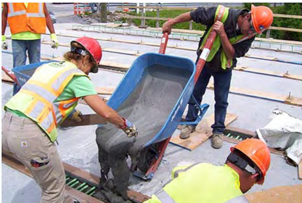
UHPC connection details make using prefabricated bridge elements simpler and more effective for accelerated bridge construction.
