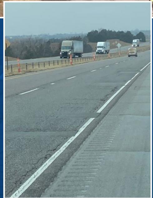
*Three TOPS countermeasures—crack attenuating mixture, highly modified asphalt, and stone matrix asphalt will be used to rehabilitate this Oklahoma interstate in 2023.*
