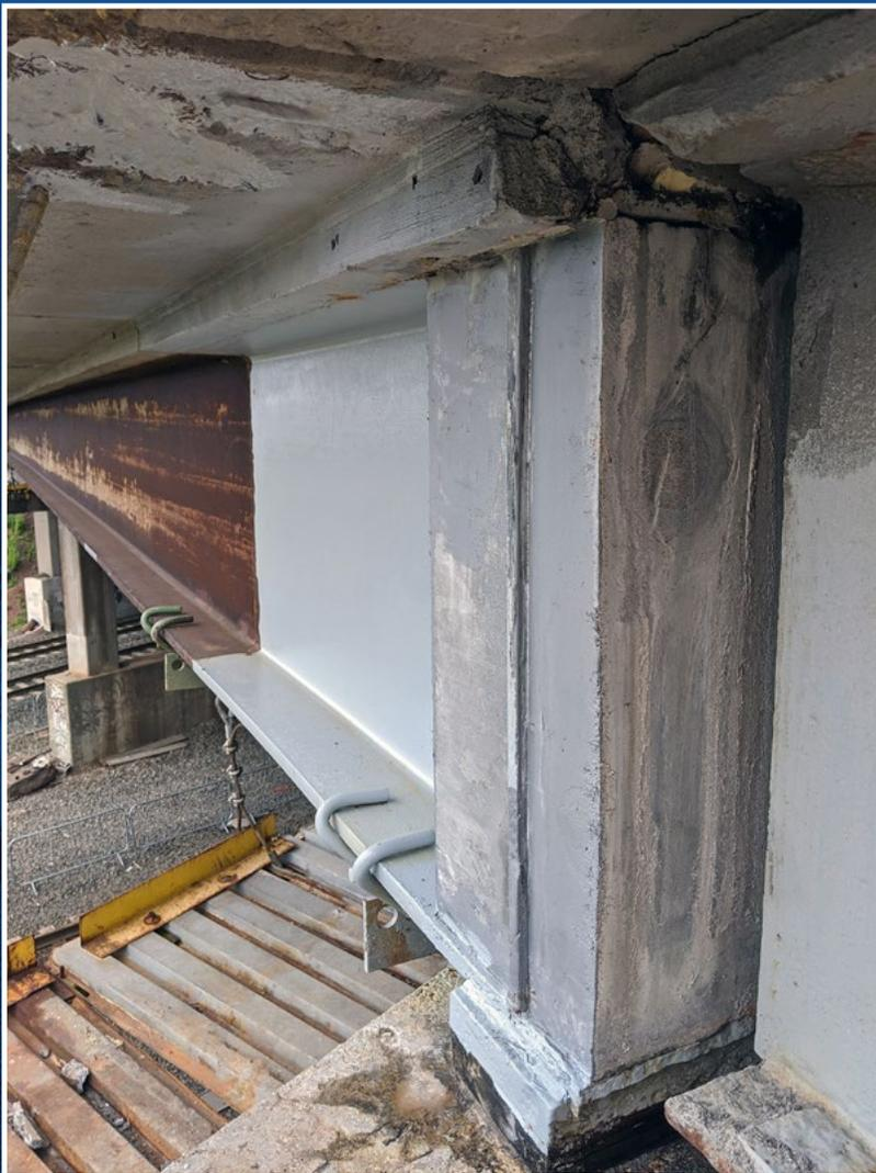
Testing of this method on a 55-year-old bridge along I-91 in New Haven, CT, revealed the UHPC repair successfully created an alternate load path through the shear connectors and UHPC. Using UHPC in this way to perform beam end repair is well adapted to working within the tight restraints of beam end supports, tight constraints of traffic control, and heavily restricted access beneath bridges.
