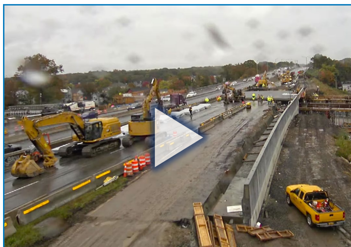
The Connecticut DOT used slide-in bridge construction for a replacement project on Interstate 95.
