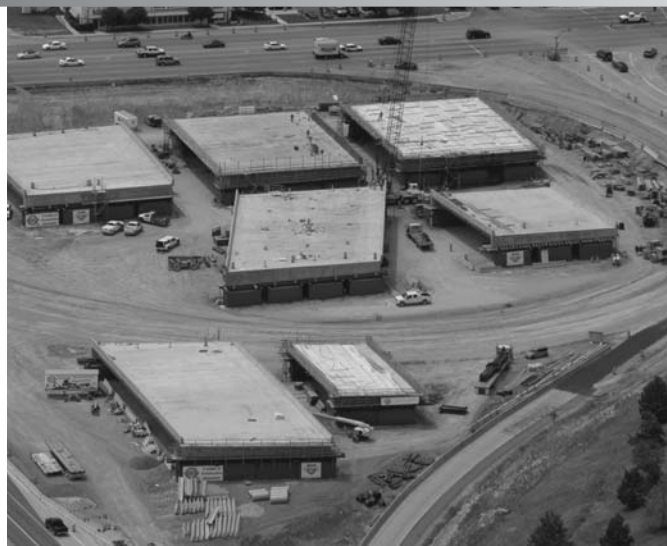
Prefabricated bridge sections at the Utah DOT’s “bridge farm” on I-80 await use on a project.
