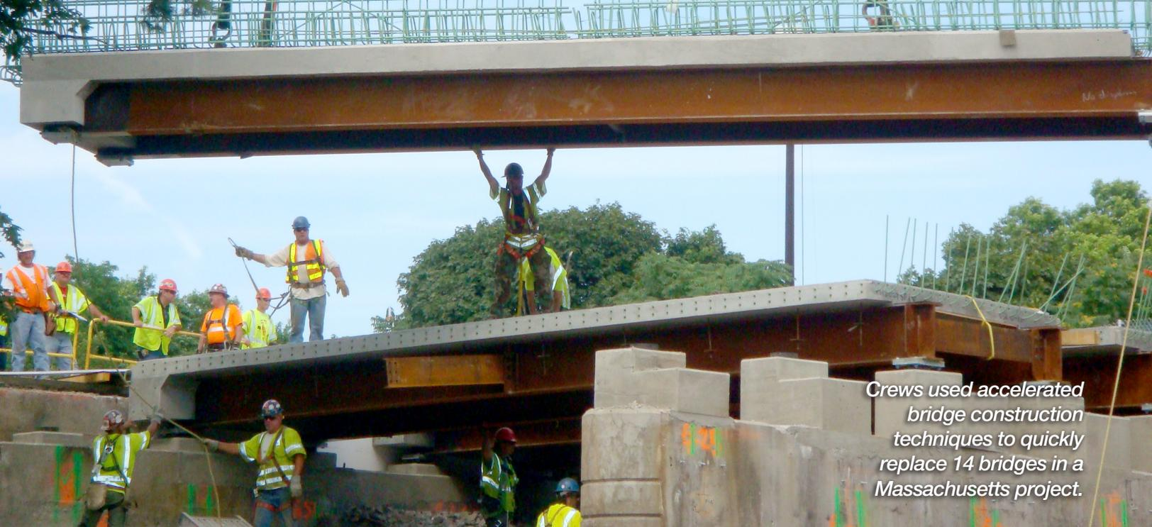
*Crews used accelerated bridge construction techniques to quickly replace 14 bridges in a Massachusetts project.*
