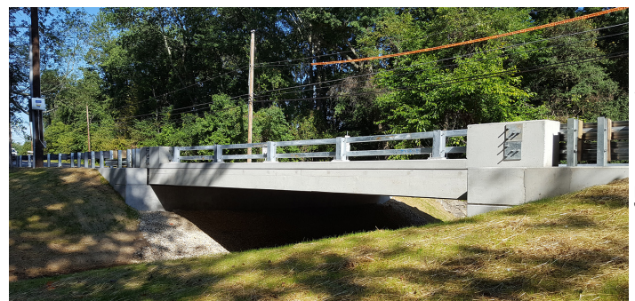
The Delaware Department of Transportation combined precast elements with UHPC connections and a UHPC overlay on an Accelerated Innovation Deployment Demonstration project.
