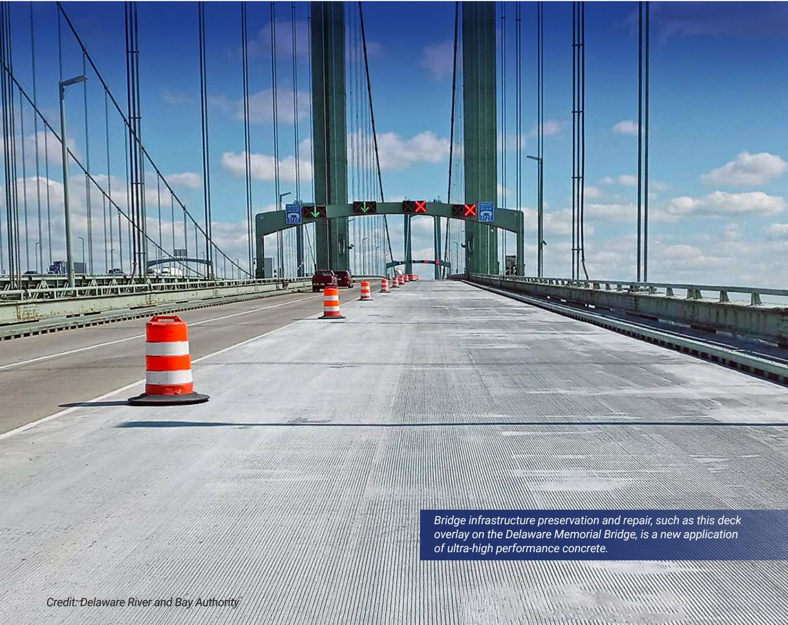
*Bridge infrastructure preservation and repair, such as this deck overlay on the Delaware Memorial Bridge, is a new application of ultra-high performance concrete.*
