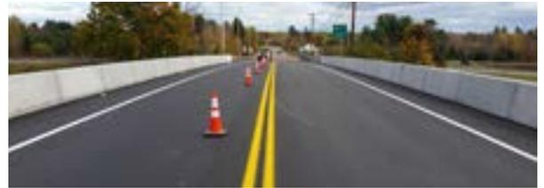
[Maine Department of Transportation \(DOT\)](#) used [STIC Incentive funds](#) for an accelerated bridge construction (ABC) project with [prefabricated concrete deck panels](#) and [ultra-high-performance concrete connections](#). The team completed the project 78 days faster than with traditional methods. The results of this project are providing lessons learned to the Maine DOT as they create statewide guidance.
