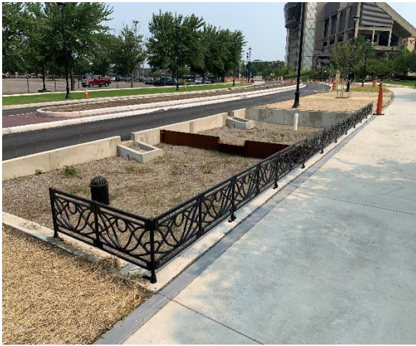
Figure 2: Mid-construction of street improvements in Youngstown, Ohio. Image courtesy of Eastgate COG.
