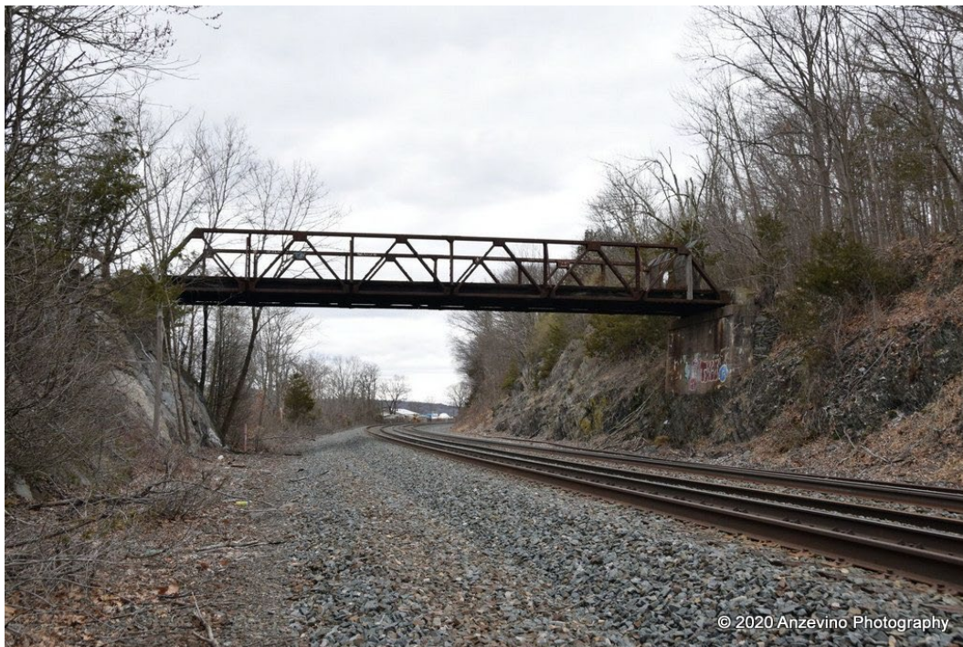
Figure 21. Pony truss bridge at the Franklin D. Roosevelt National Historic Site.
