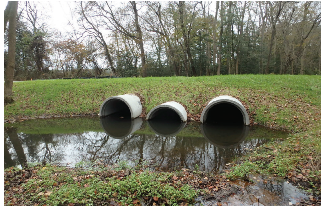
DeL DOT Pipe Culvert Bundle.
