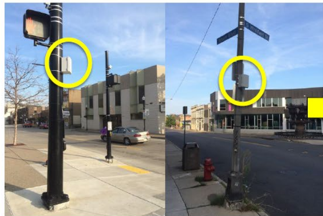
Low-cost automatic vehicle identification (AVI) sensors
